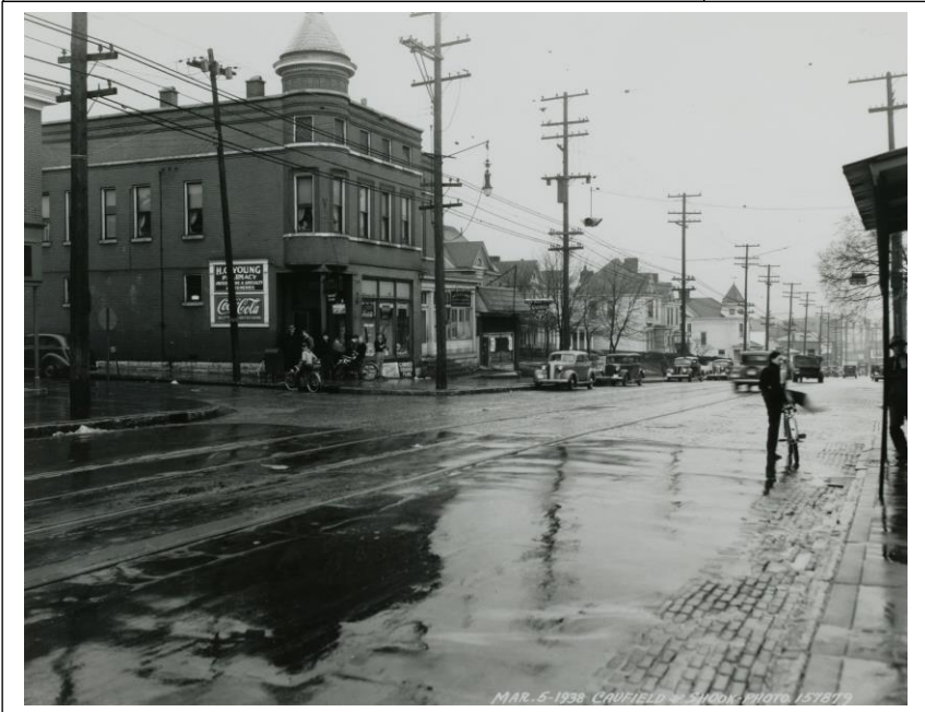
10 S.W. Corner of Frankfort Ave. and Pope St., March 5, 1938
