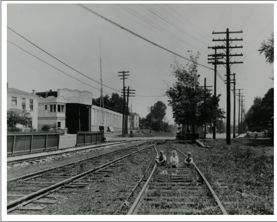
33 Railroad tracks and New Main University of Louisville Photographic Archives
